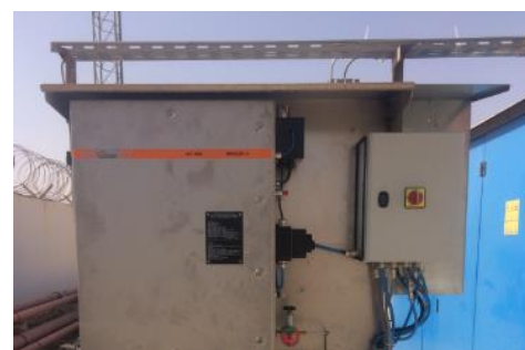
Figure 2. Picture of the energyMEDOR in hazardous area ATEX zone 1
