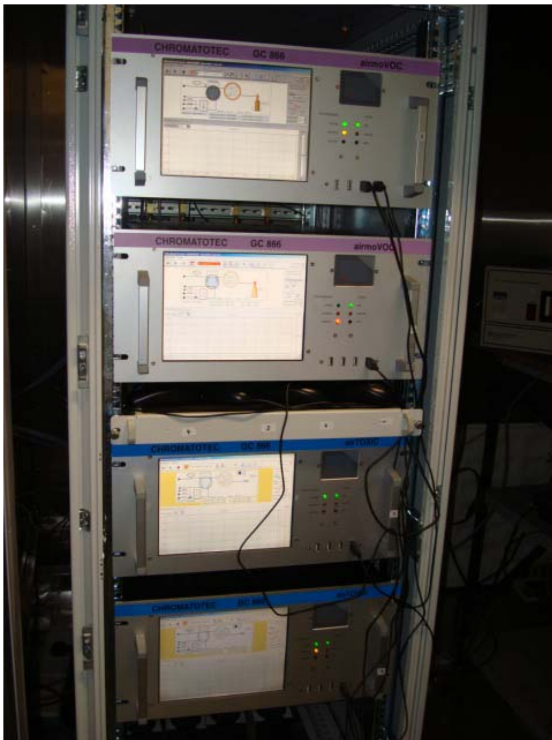
Figure 16: Photograph showing all four CAMs in operation, located in NPL's environmental chamber.
